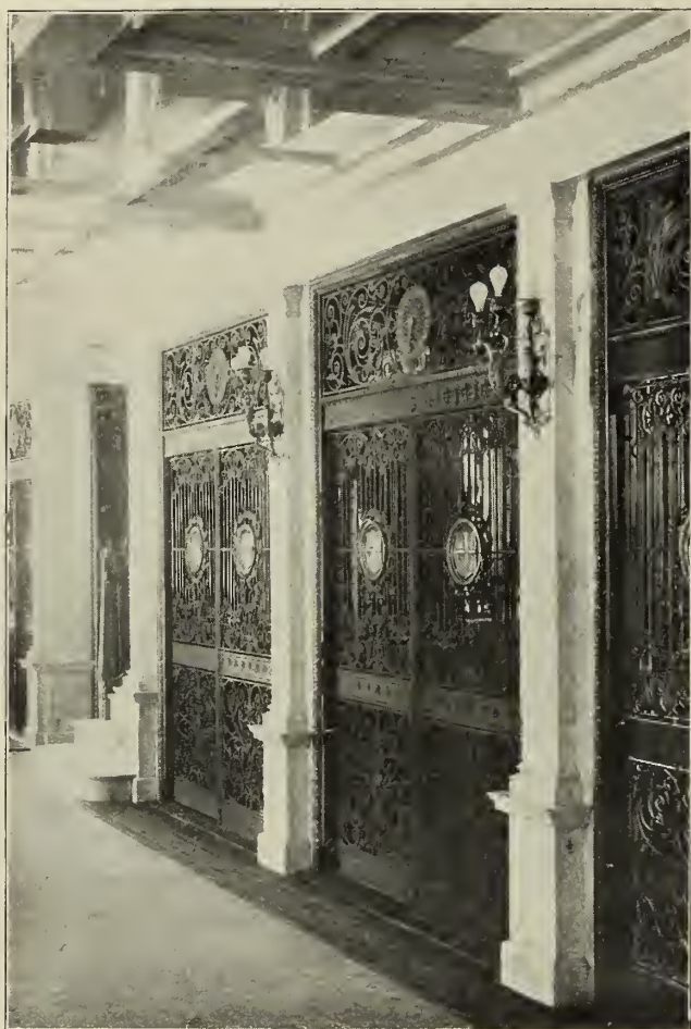
A.—ELEVATOR INCLOSURE, OLD COLONY BUILDING, CHICAGO. Wrought Iron, Hammered Leaf Work, Bower-Barffed. Rails and Coat of Arms in Bronze.
